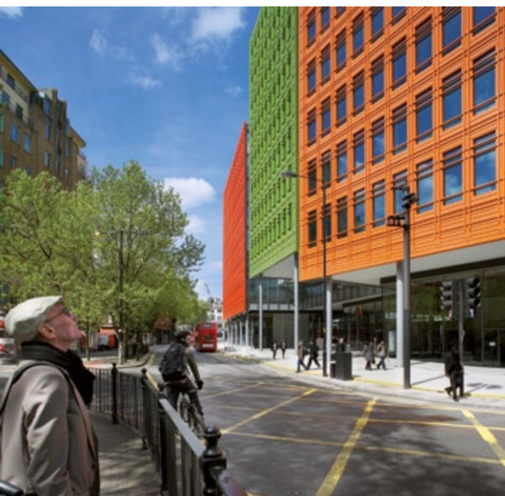
NBK KERAMIK: 140,000 ceramic elements in six different colours: RAL 070 70 80, RAL 050 50 70, RAL 050 50 78, RAL 000 75 00, RAL 110 60 50 and RAL 7035 Light grey.
